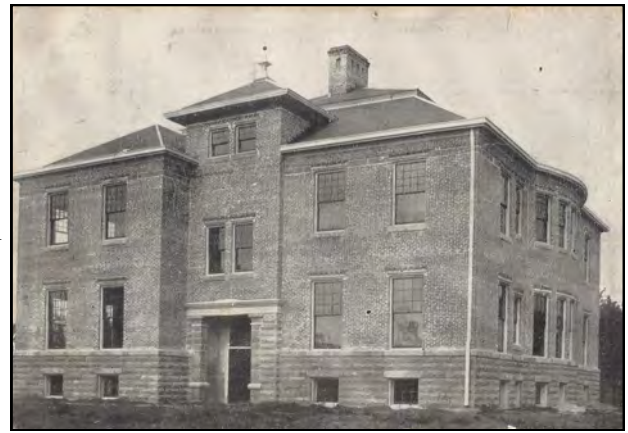
Lebo's first brick school building built in 1907 at the cost of $13,000.
